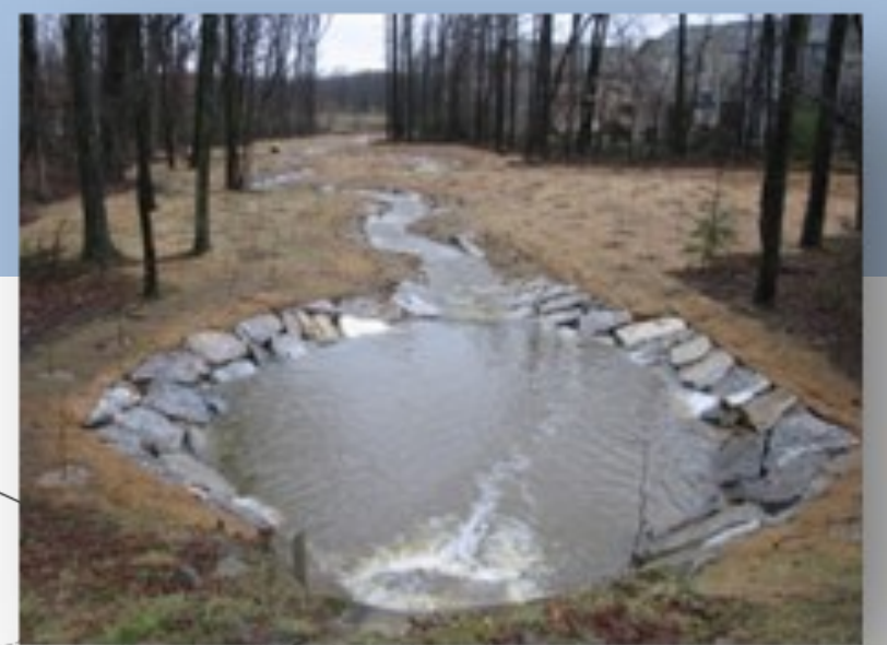
Stilling basin (plunge pool)
