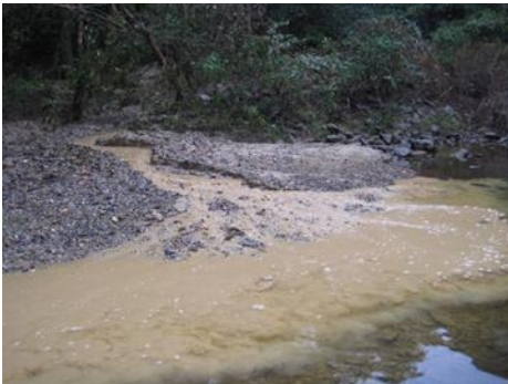
Construction sediment in creek ☹
